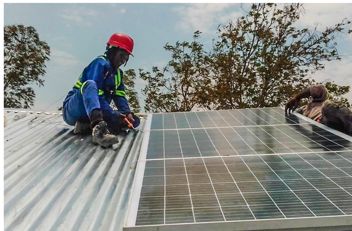
Installing solar panels on the school
