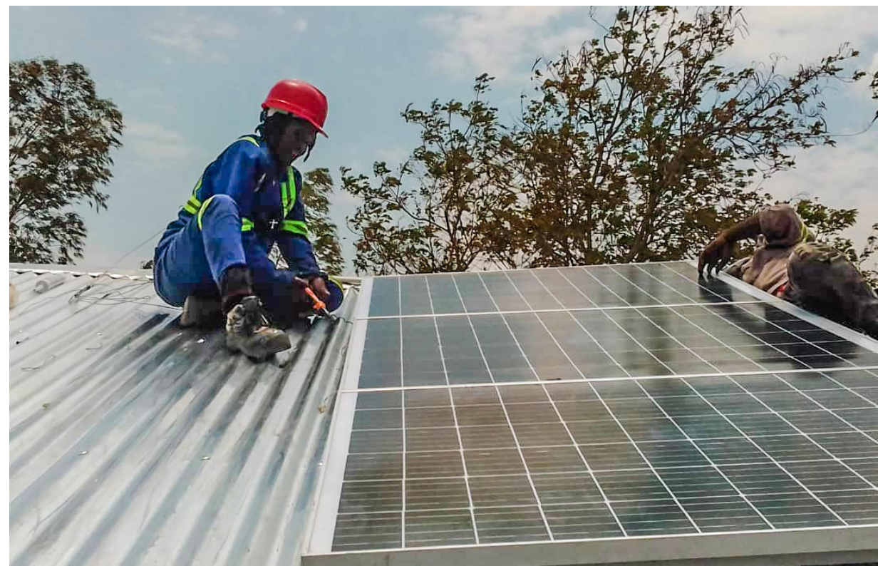
Installing solar panels on the school
